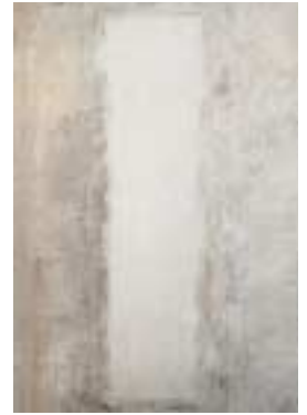
R20/20 repair of concrete surfaces
